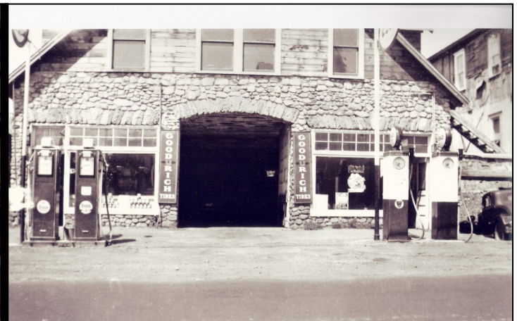
Right: Cresco Garage after the apartment was added
